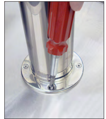
FIG. 3. Secure the draft standard to the countertop.
