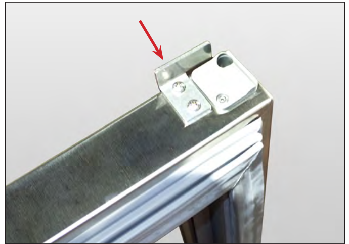
FIG. 4. Doorstop bracket installed on door.
